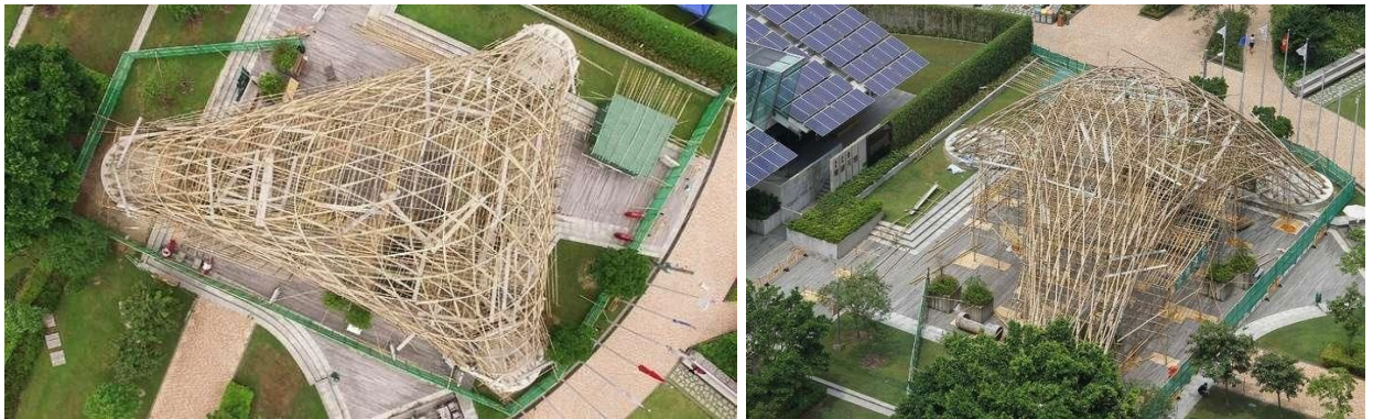
Fig.2 shows the self-supporting bamboo structure from locally sourced poles bent together to form a lightweight durable framework.
